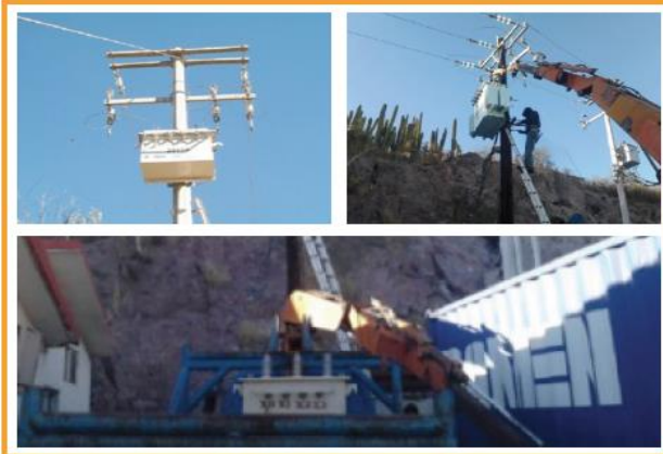
Maintenance to existing installations for Mine Multatos in Sonora
